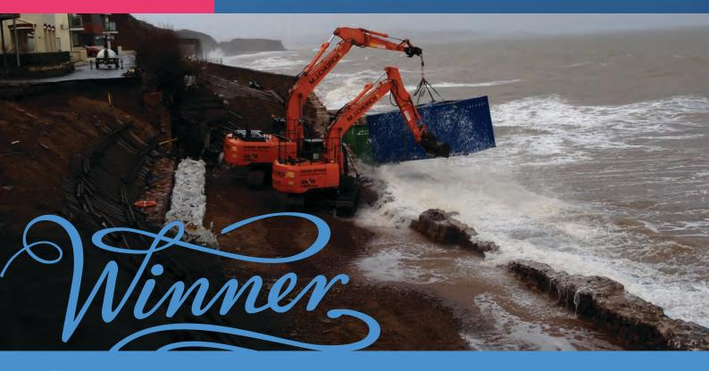
Emergency repairs at Dawlish presented many challenges for Network Rail, including the need to stabilise a massive sea cliff after failure caused by the intense rainfall in the storm conditions. The project team's innovative solution - deliberately initiating a landslide was crucial in getting the line open again, as well as earning the team the APM's Project of the Year award.
