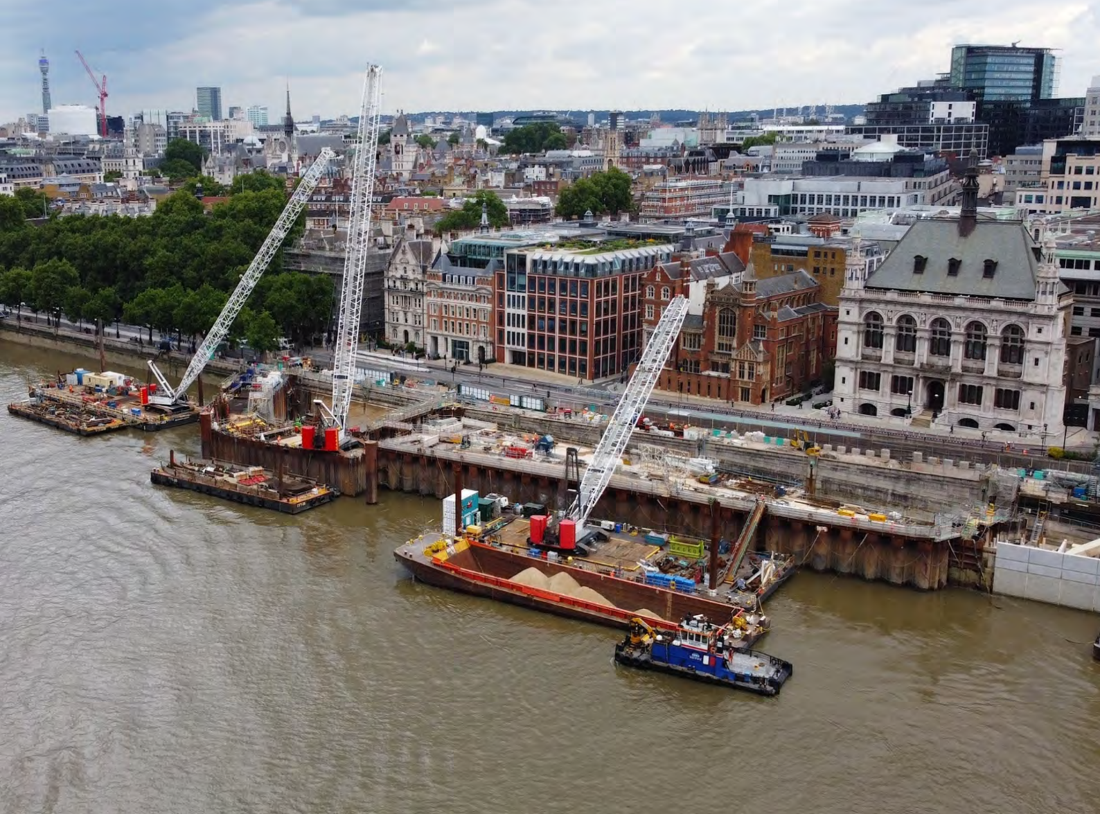
Image: London Tideway project near Blackfriars bridge, aerial view; Steve Bateman via Getty Images
